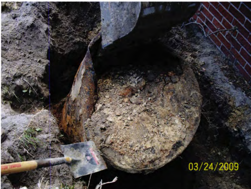
Picture 4: UST 156 Laurel Bay Blvd.-2 being removed from the excavation.
