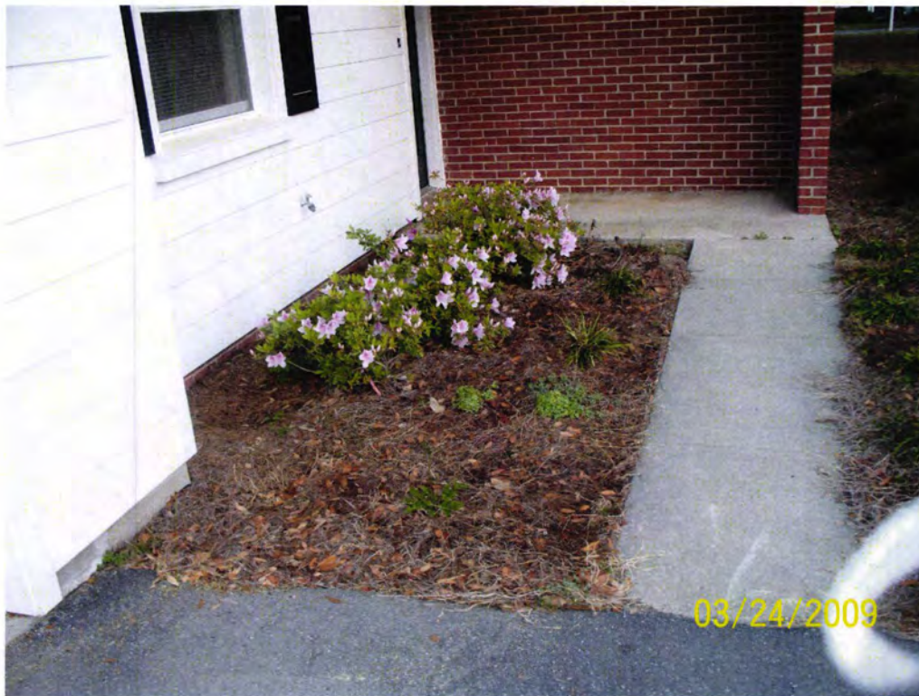
Picture 1: Location and condition of UST 156 Laurel Bay Blvd-1 prior to removal of the tank.
