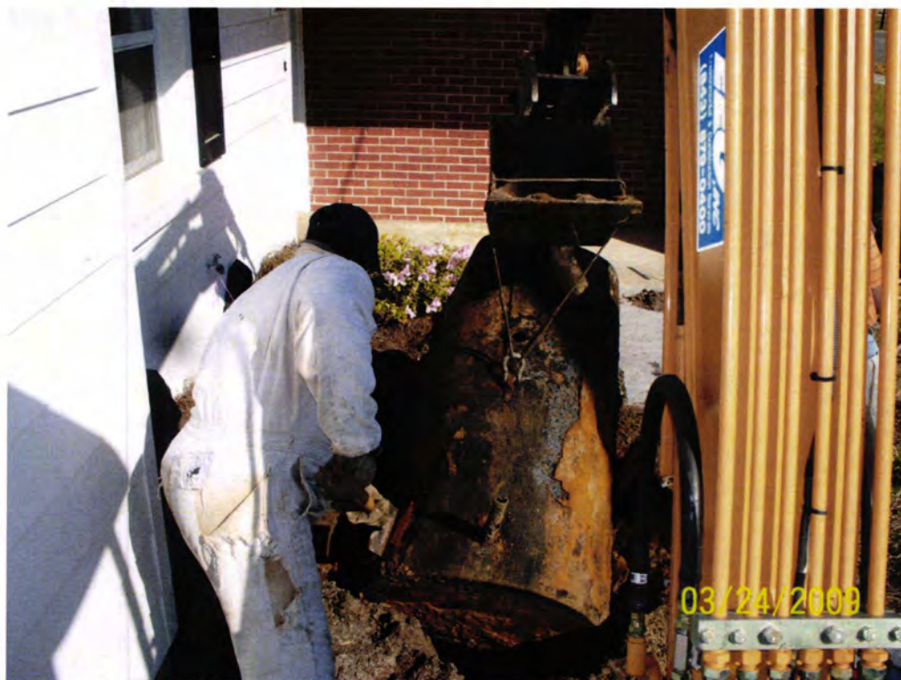
Picture 2: UST 156 Laurel Bay Blvd-1 being removed from the excavation.
